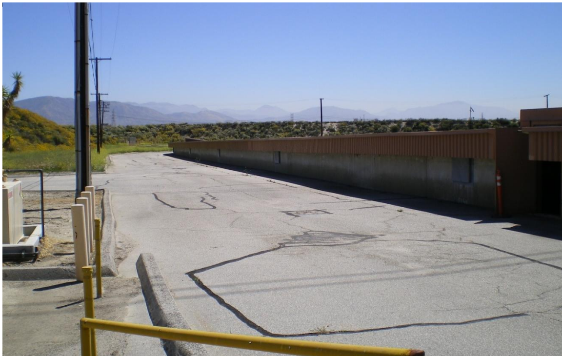
Photo B. Reservoir profile from north side looking easterly.
