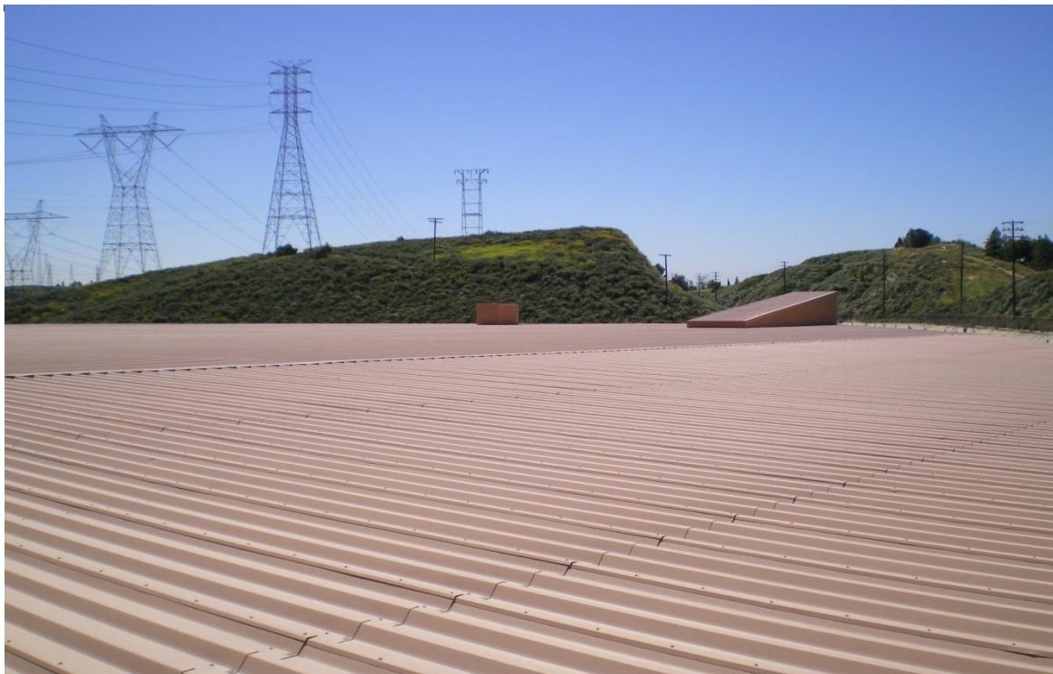
Photo D. Reservoir corrugated metal roof; looking southerly.
