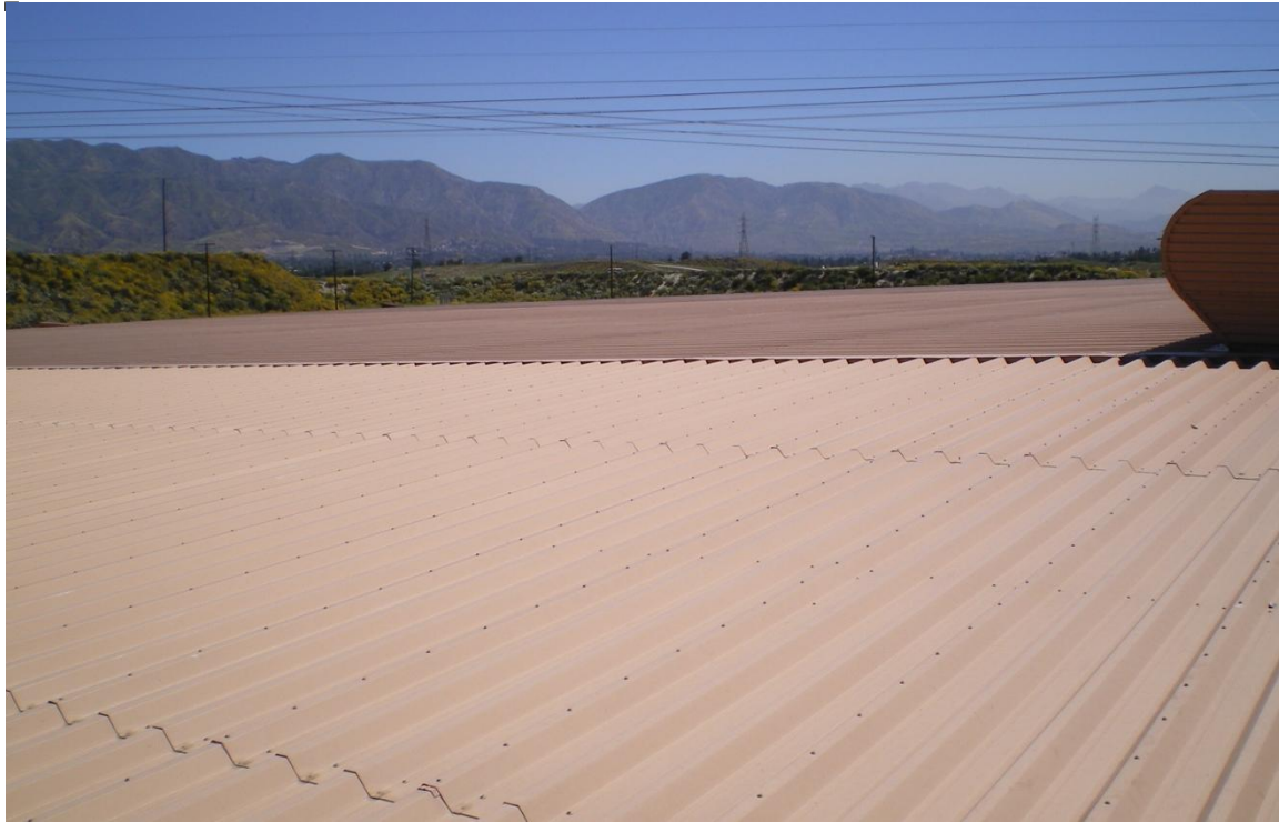
Photo E. Reservoir corrugated metal roof; looking northeasterly.
