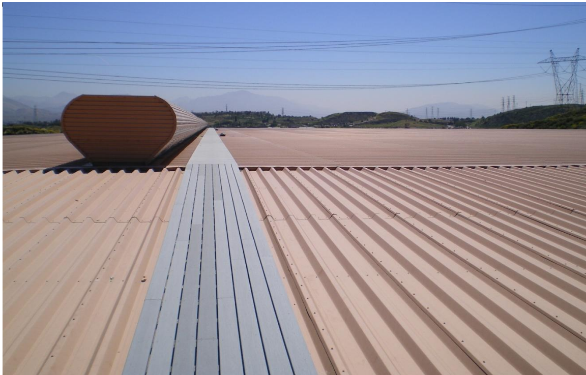
Photo F. Reservoir corrugated metal roof; looking easterly.
