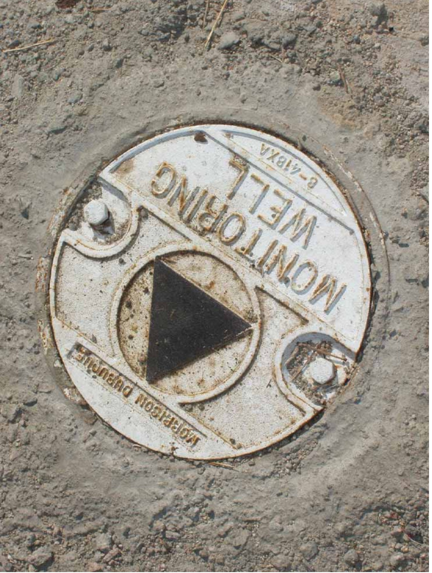
B-11 Rock Coring (Not A Monitoring Well) On Top Of Terminal Hill
