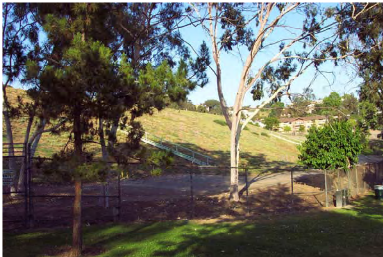
Figure 2-4 Silver Lake Reservoir Dam
