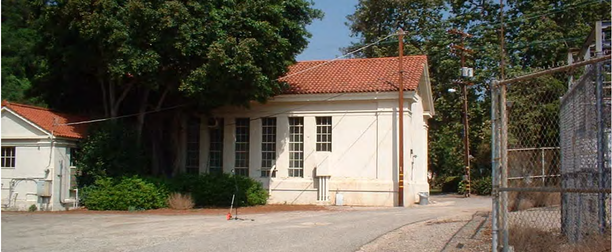
Figure 11: Franklin Canyon Power House
