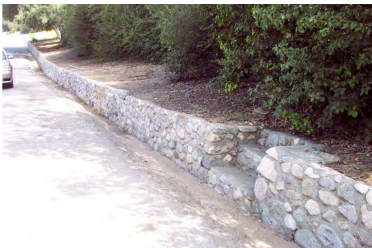
Figure 2-13 Stone Retaining Walls
