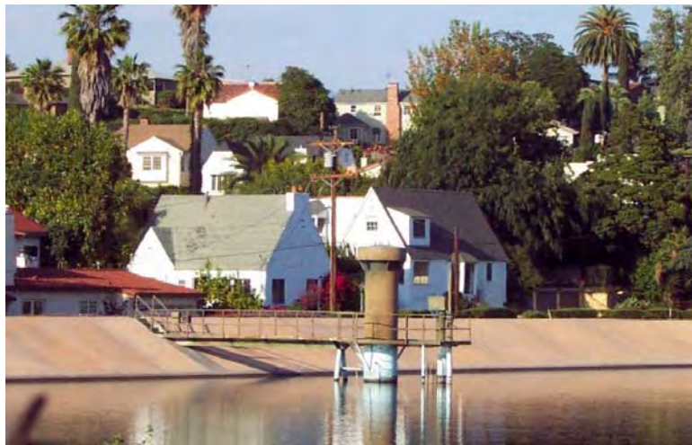
Figure 2-3 Ivanhoe Reservoir Inlet Tower
