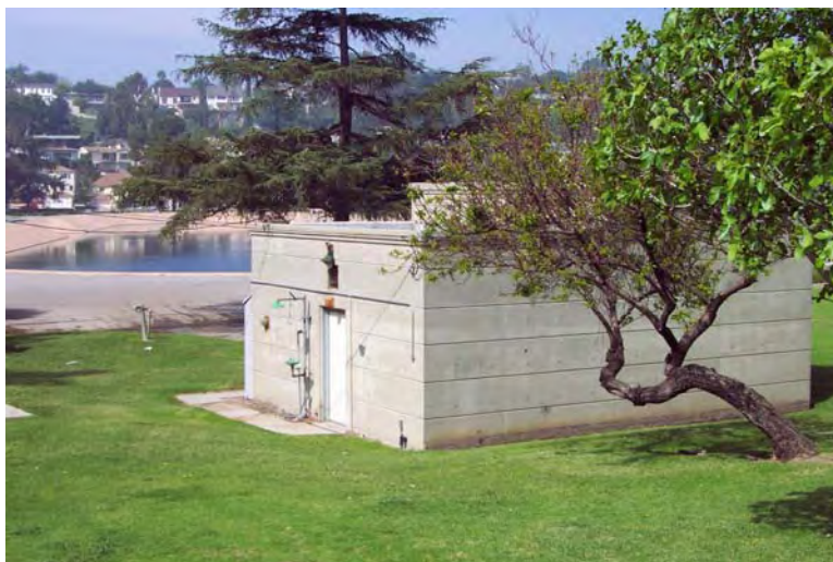
Figure 2-12 Ivanhoe Chlorination Station
