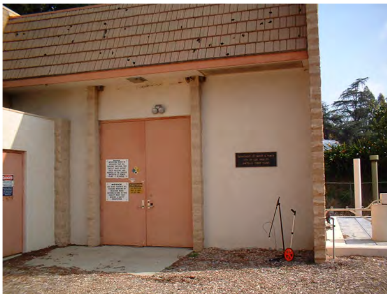
Figure 10: Sawtelle Power Plant (inoperative)
