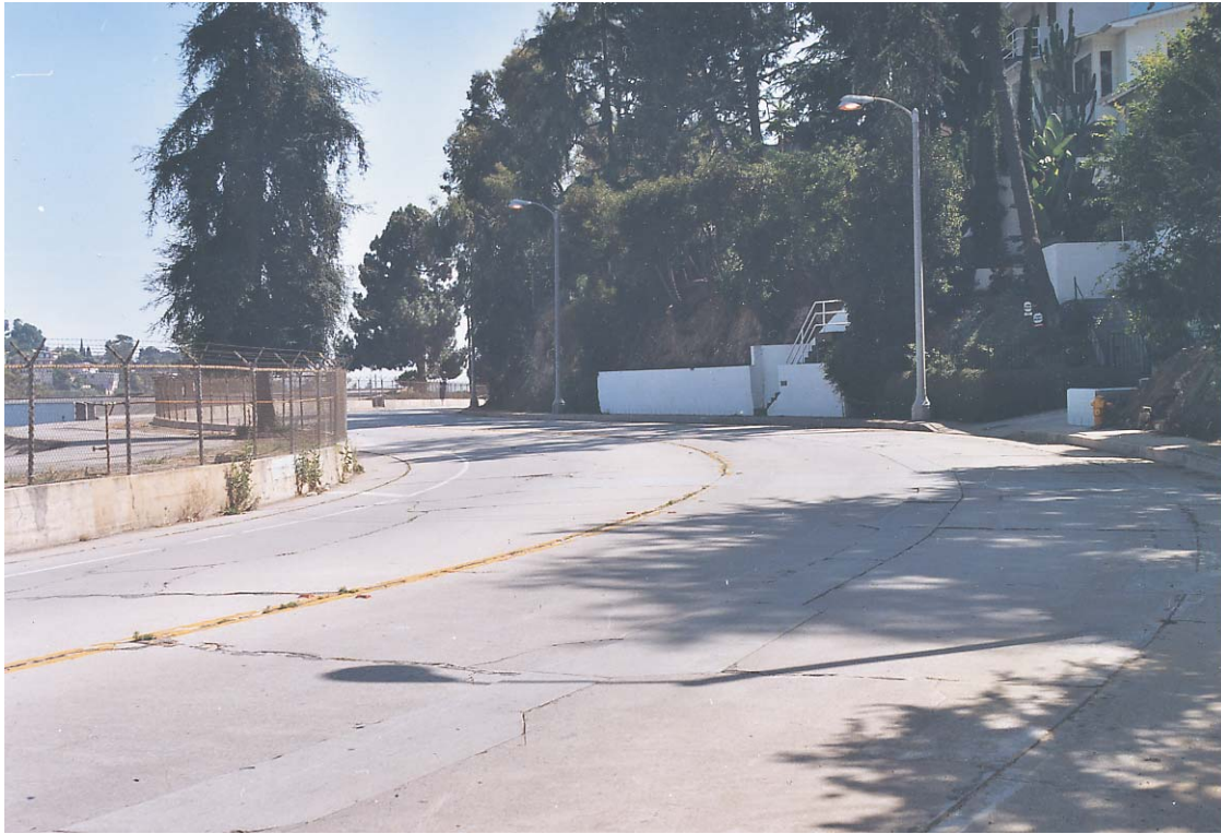
Photo 9. Existing view looking south on West Silver Lake Drive toward the location of the bypass pipeline receiving pit.
