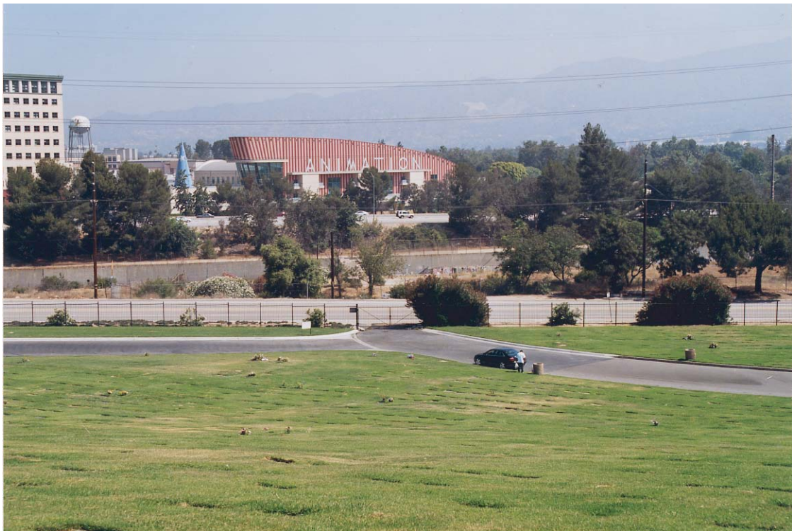
Photo 6. Existing view looking south across proposed hydroelectric plant site from the area near Greenwood Way in Forest Lawn Memorial Park.
