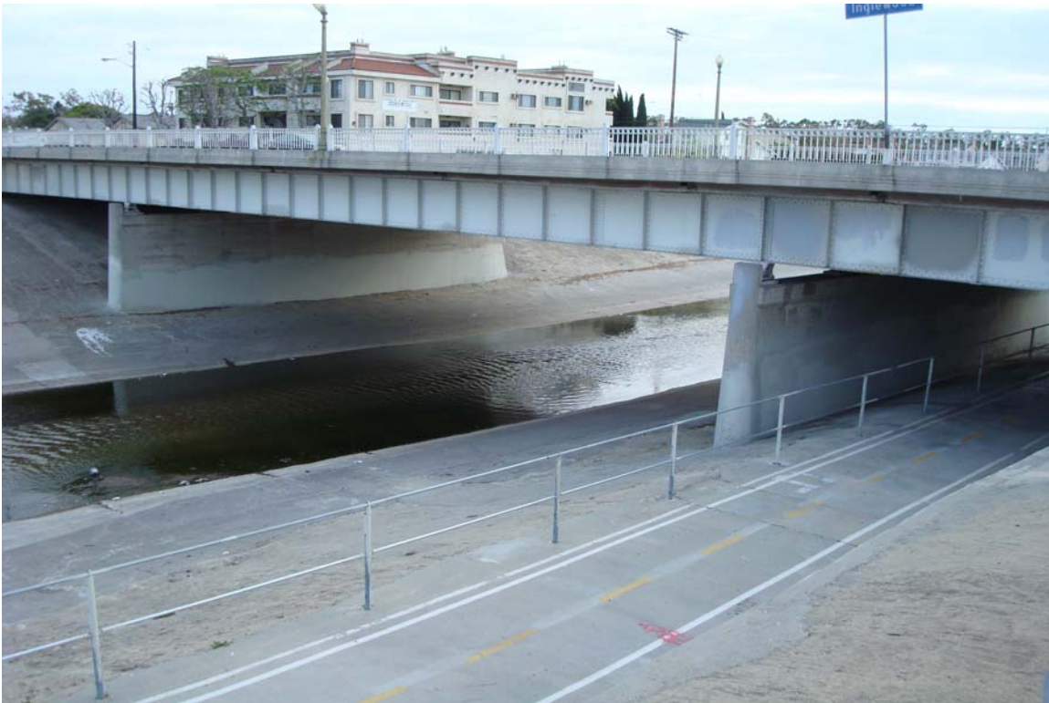
Photograph 7. West-facing view of the Inglewood Boulevard Ballona Creek Bridge
