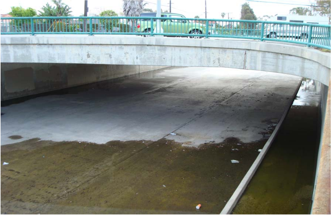
Photograph 6. West-facing view of the Inglewood Boulevard Centinela Creek Bridge.
