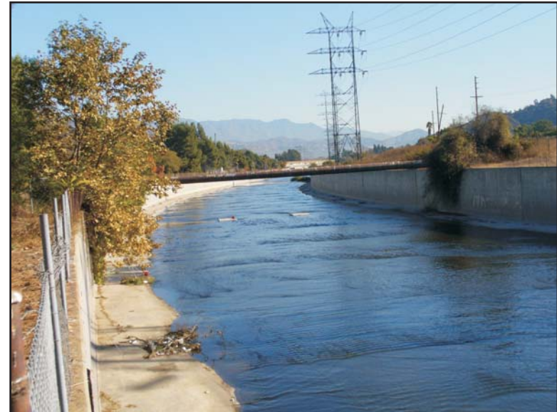
12. View northeast at Los Angeles River
