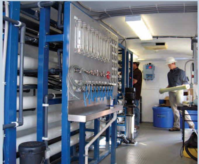
Membrane filters installation
