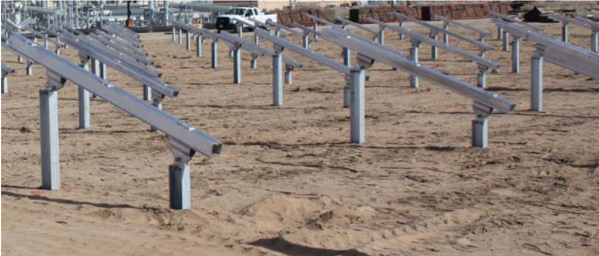
Figure 5 Owens Lake Solar Demonstration Project – Pile Driven Pier Foundations
