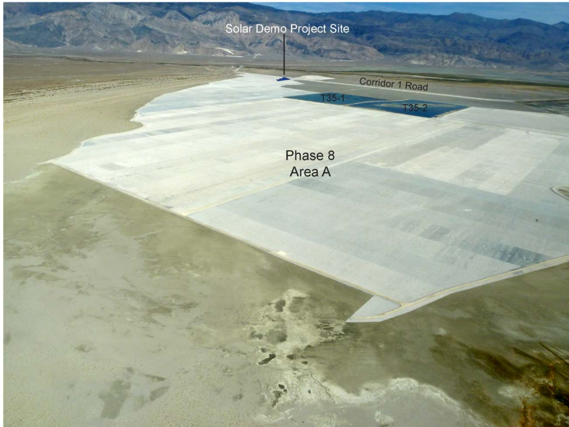
Figure 8 Aerial View of Solar Demo Project Site (Looking East)
