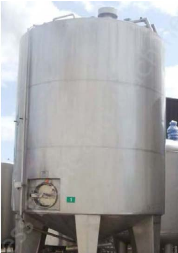
Typical Hydrogen Peroxide Storage Tank
