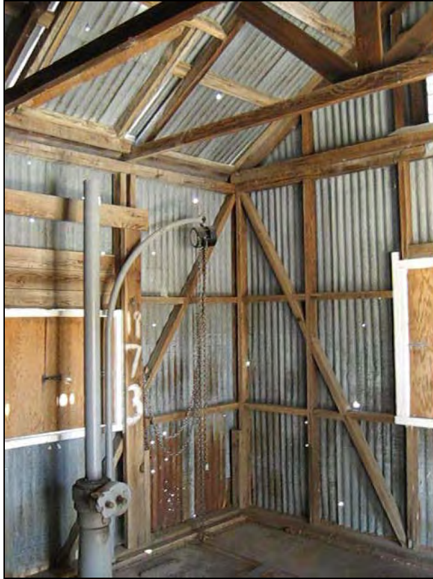
Figure 7.6 Interior of the Mono Gate One structure.
