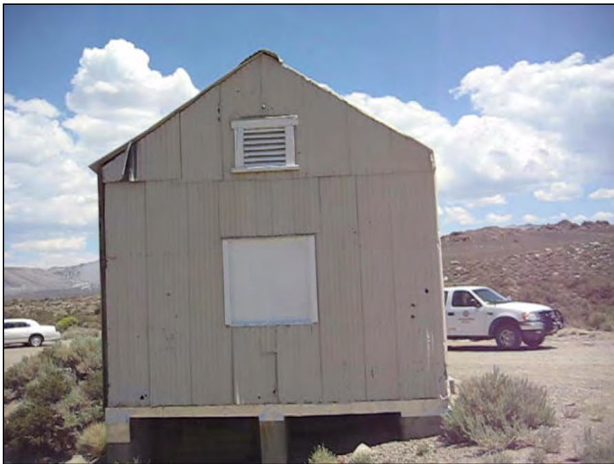
Figure 7.3 The west elevation of the Mono Gate One structure.
