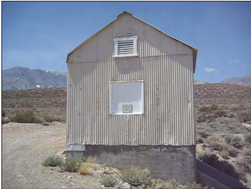
Figure 7.5 The east elevation of the Mono Gate One structure.
