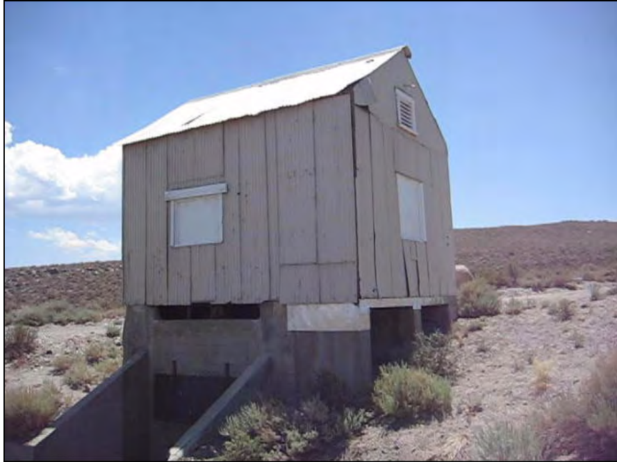
Figure 7.4 The north and west elevations of the Mono Gate One structure.
