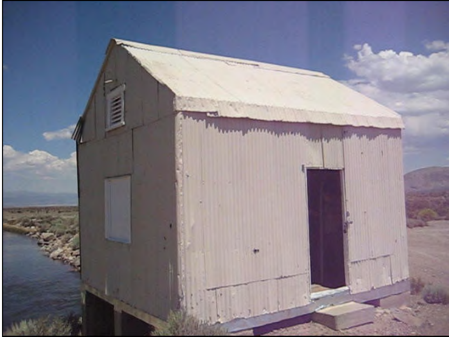
Figure 7.2 The south and west elevations of the Mono Gate One structure.
