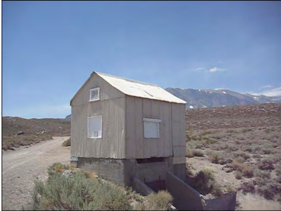
Figure 7.1 The north and east elevations of Mono Gate One structure.
