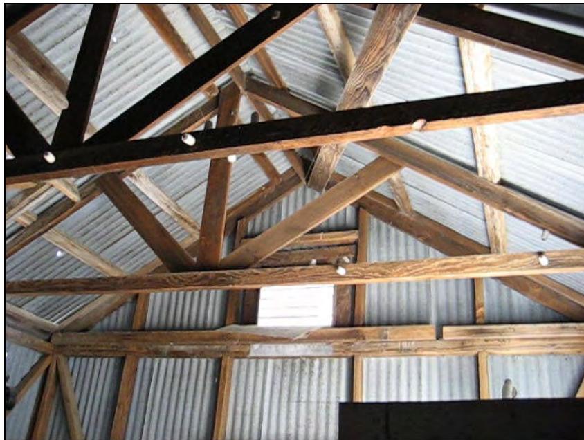
Figure 7.7 The interior of the Mono Gate One structure.
