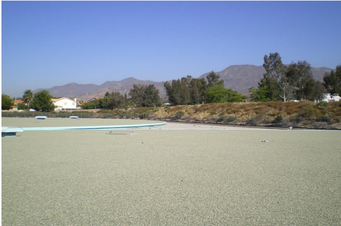
Photo A. Tank roofs, looking west.
