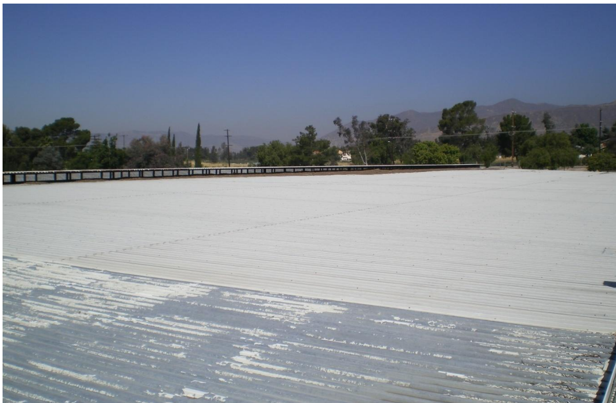
Photo D. Reservoir roof, looking west.
