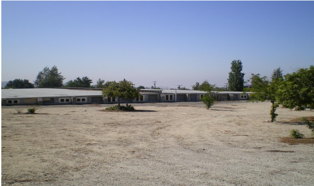
Photo C. Northwest side of reservoir, looking south.
