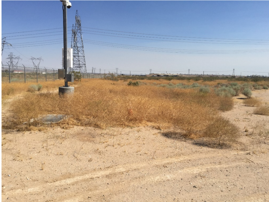
View toward the northwest corner of the Adelanto Switching Station and a planned temporary use area near existing high voltage transmission lines. Image #3487. June 11, 2020.
