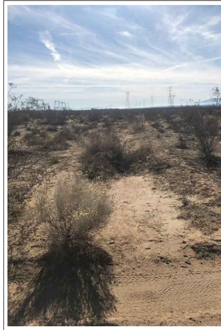
Photo B - View of Drainage 1 from the northern edge of the Project site with the Adelanto Converter Station in the background.
