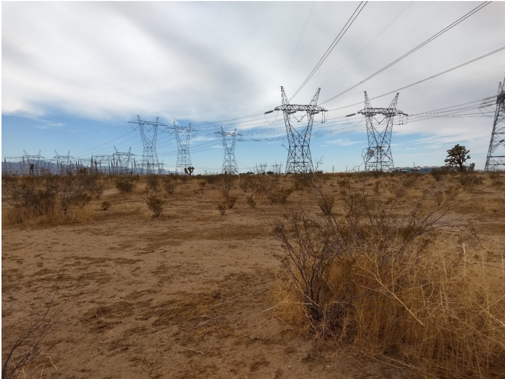
PHOTO 1 PHOTO POINT LOCATED IN THE NORTHEASTERN PORTION OF THE PROJECT SITE, FACING SOUTHWEST.
