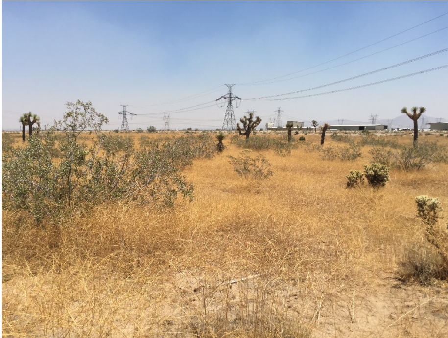
View toward the northeast near the center of the Adelanto Switching Station and a planned temporary use area near existing high voltage transmission lines. Image #3510. June 11, 2020.
