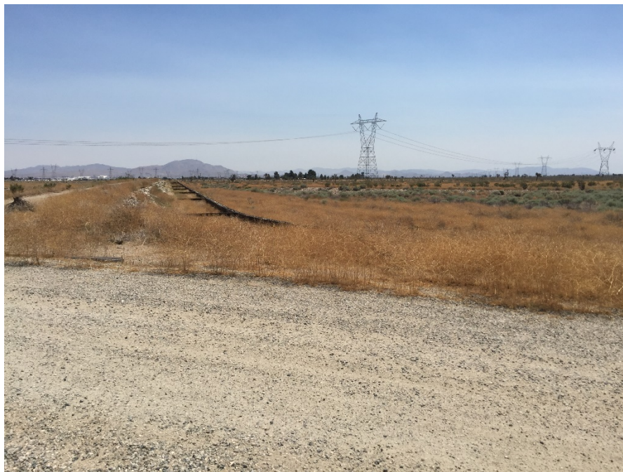
View toward the west from the southeast corner of the Adelanto Switching Station and a planned temporary use area near existing high voltage transmission lines. Image #3505. June 11, 2020.
