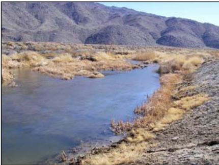
Below Blackrock Return Ditch at 50 cfs.
