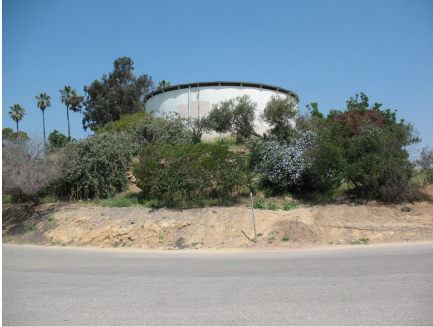
Photo 9. Photo depicting the existing water tank and surrounding habitat on the hilltop by Elysian Fields. Photo facing north.
