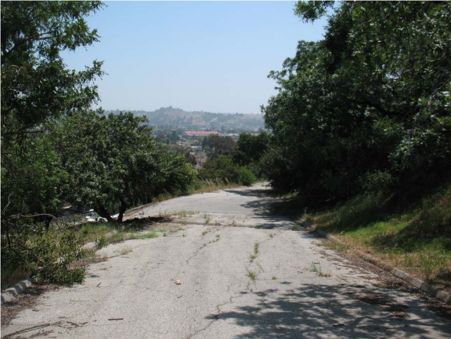
Photo 2. Photo of proposed recycled water pipeline route between Stadium Way and the proposed location for a new recycled water pumping station. Photo facing east.
