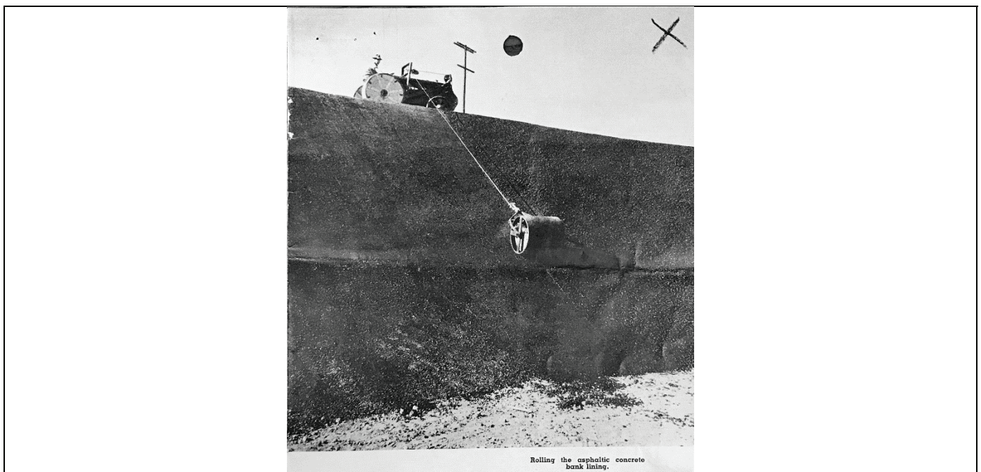
Figure 4. Photo demonstrating roller compaction at De Soto Reservoir, 1942. (DWP Record Center)
