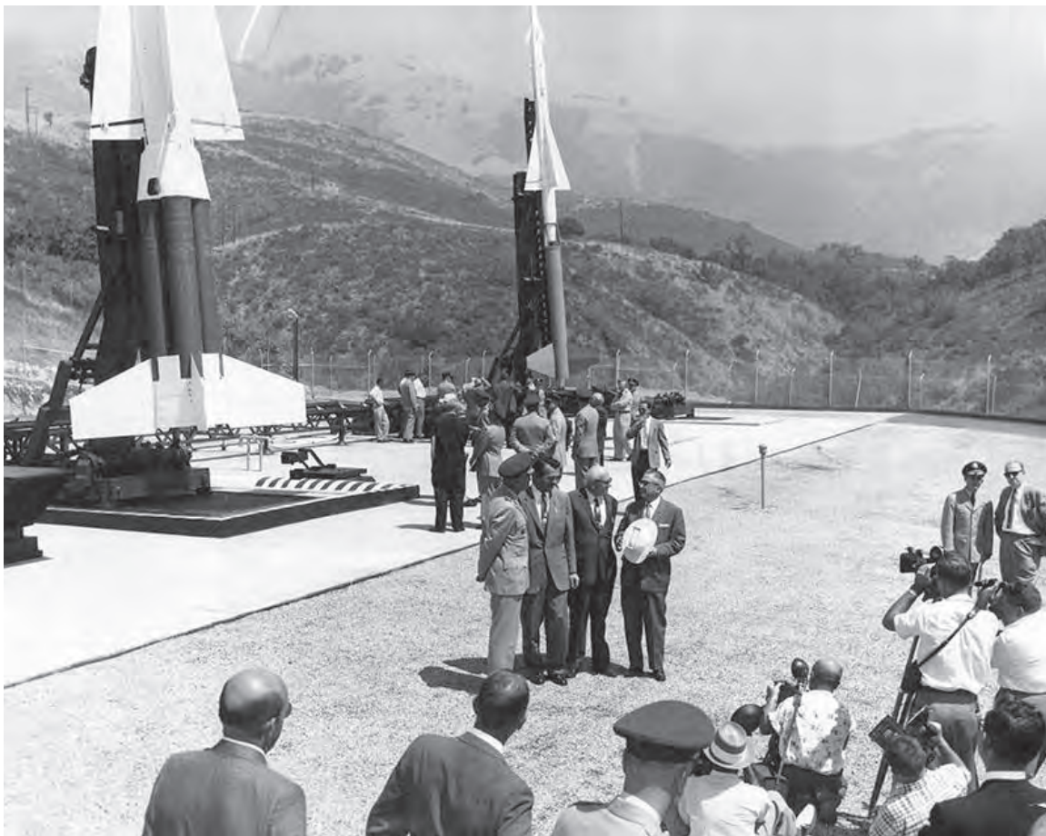
Figure 6. Oat Mountain Nike-Hercules Base in Chatsworth California., looking north, 1958 (Los Angeles Public Library LAPL00114029)
