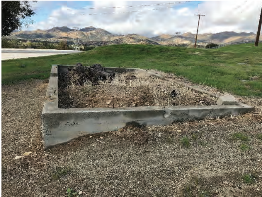
Figure 12. Board-formed concrete building foundation, looking southwest. March 14, 2018. (IMG1670)
