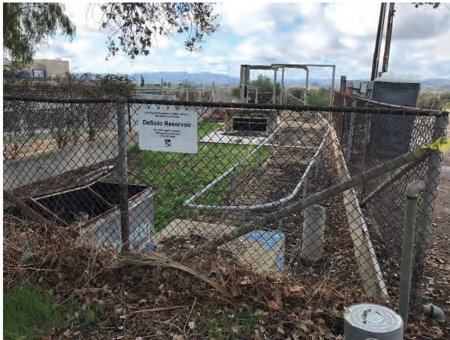
Figure 14. Meteorological Station, looking southwest. March 14, 2018. (IMG1677)
