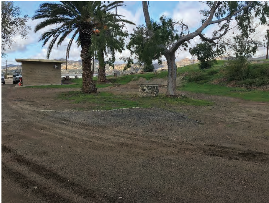
Figure 13. Well features and chlorination outbuilding, looking west. March 14, 2018. (IMG1674)
