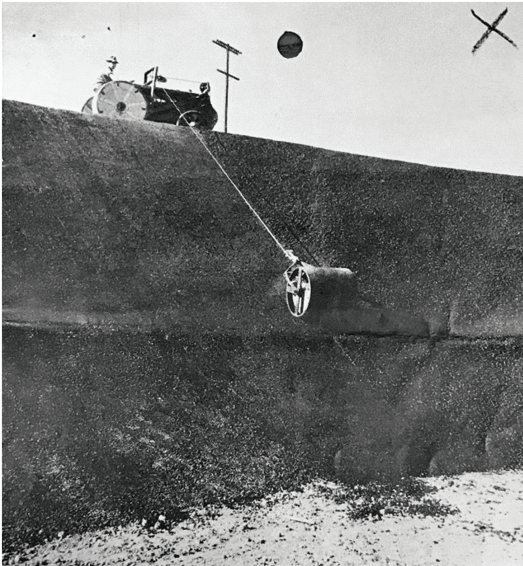
Figure 7. Photo demonstrating roller compaction technique at De Soto Reservoir, 1942. (LADWP Record Center)
