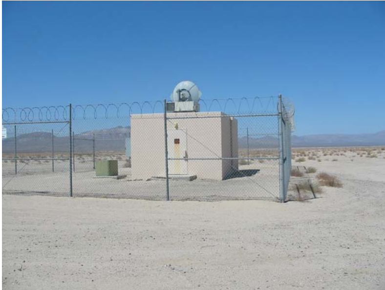
Figure 1-2 Existing Site Conditions – Terminal Building
