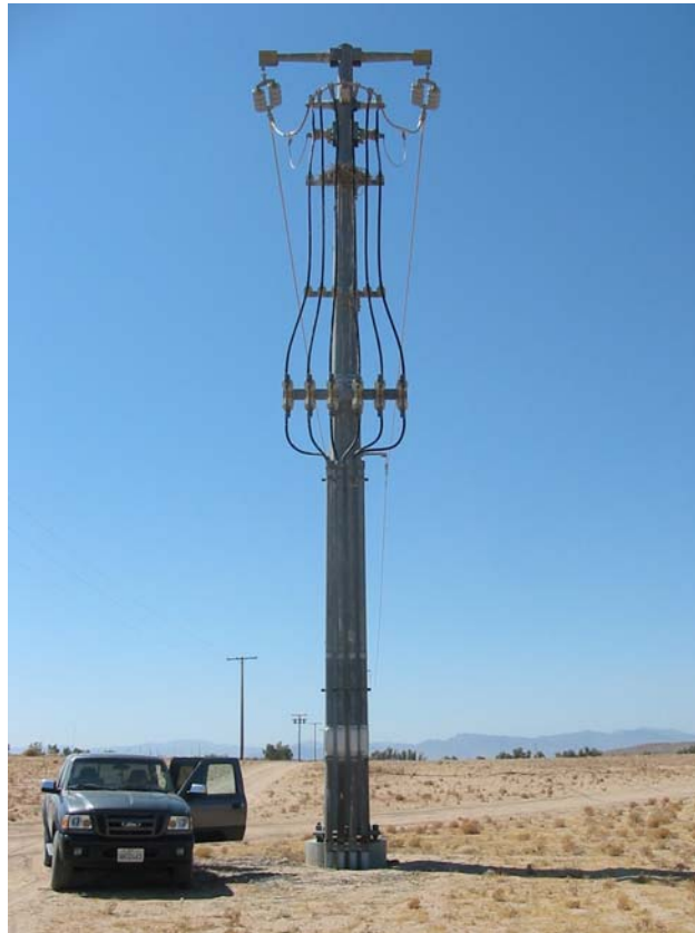
Figure 1-3 Existing Site Conditions – Terminal Pole
