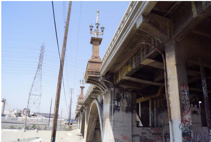
Figure 2. Olympic Street Bridge-view of Decorative Light Fixtures
