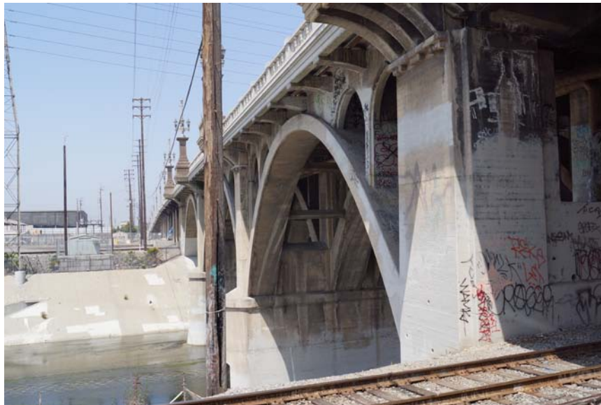
Figure 1. Olympic Boulevard Bridge
