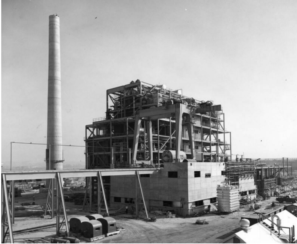
Figure 1. Units 1 and 2 under construction, 1953 (DWP Photo Collection, Los Angeles Public Library)
