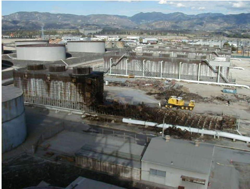
Figure 11. Units 1 and 2 cooling towers being demolished, 2000 (On file at LADWP)
