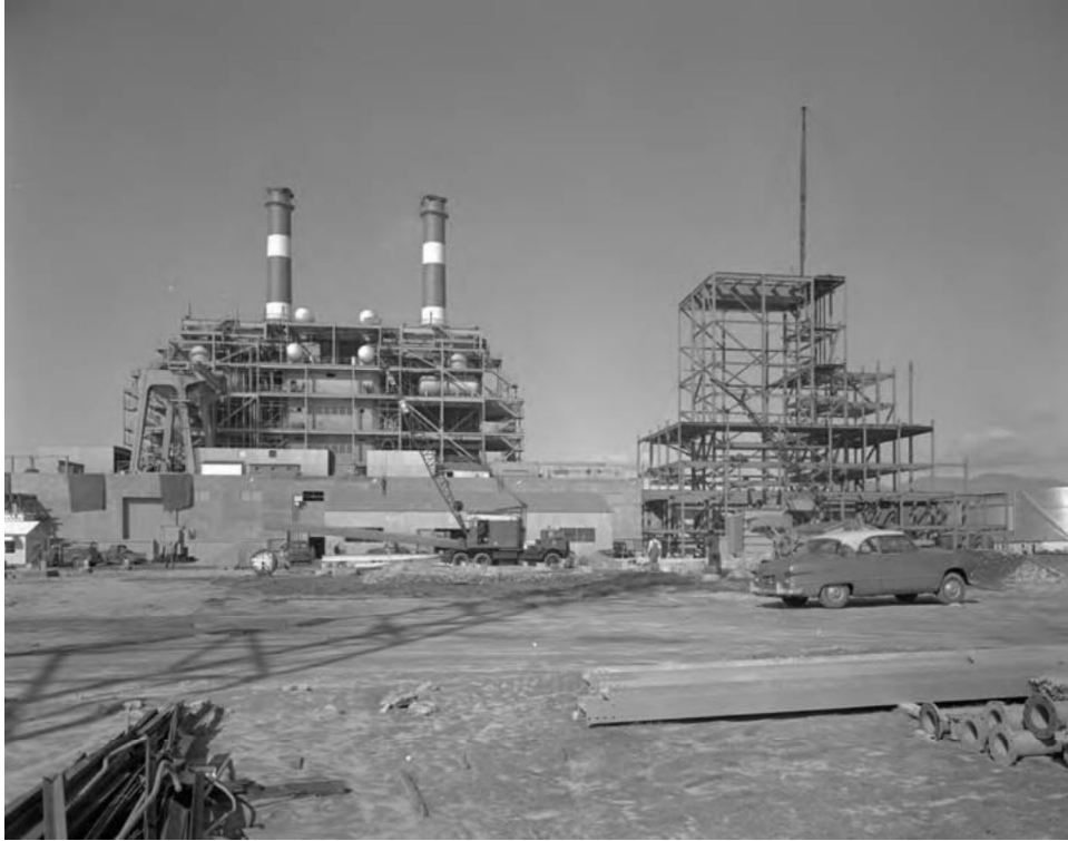
Figure 2. Units 3 and 4 under construction, 1954 (DWP Photo Collection, Los Angeles Public Library)
