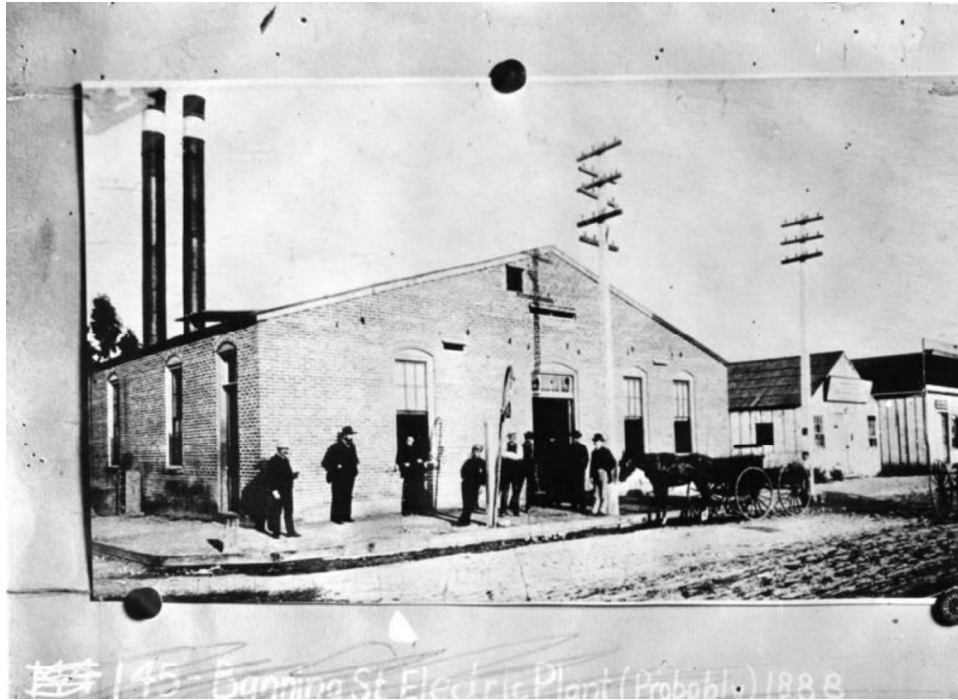
Figure 5. Banning Street Electrical Plant, circa 1888 (Security Pacific National Bank Collection, Los Angeles Public Library)
