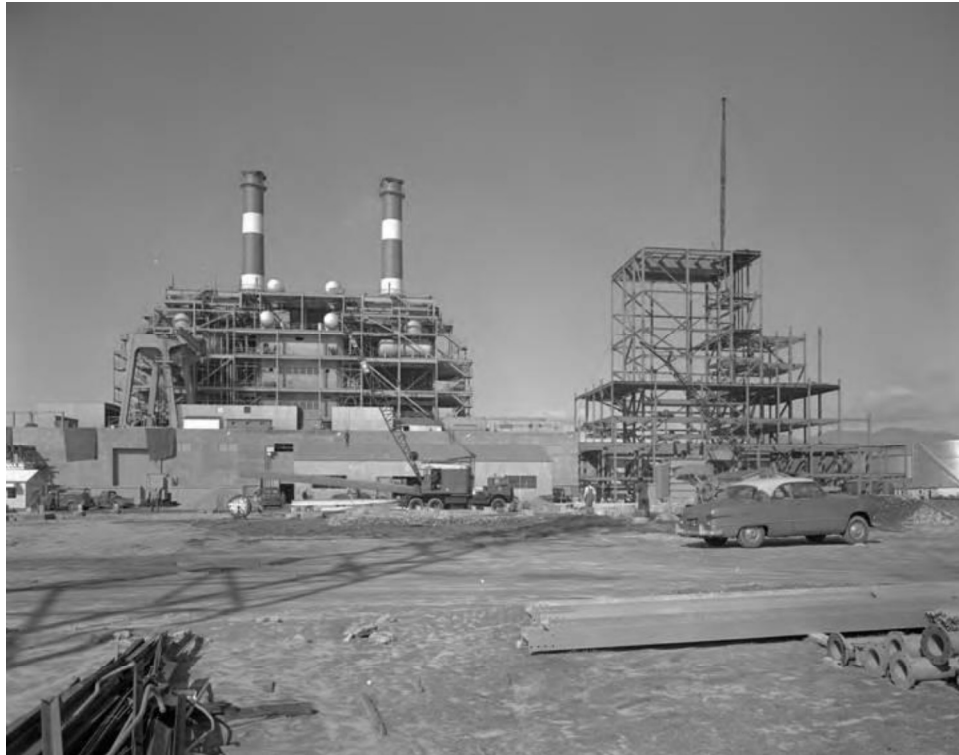
Figure 9. Units 3 and 4 under construction, 1954 (DWP Photo Collection, Los Angeles Public Library)
