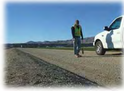
Electromagnetic (EM) utility location (archive photo)
