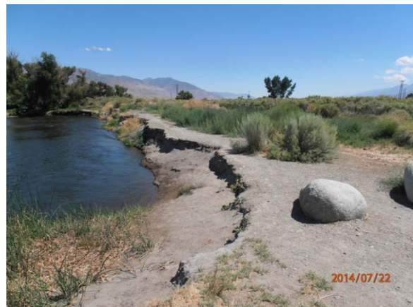
Hwy 6 & Owens River N Parking, July 2014
