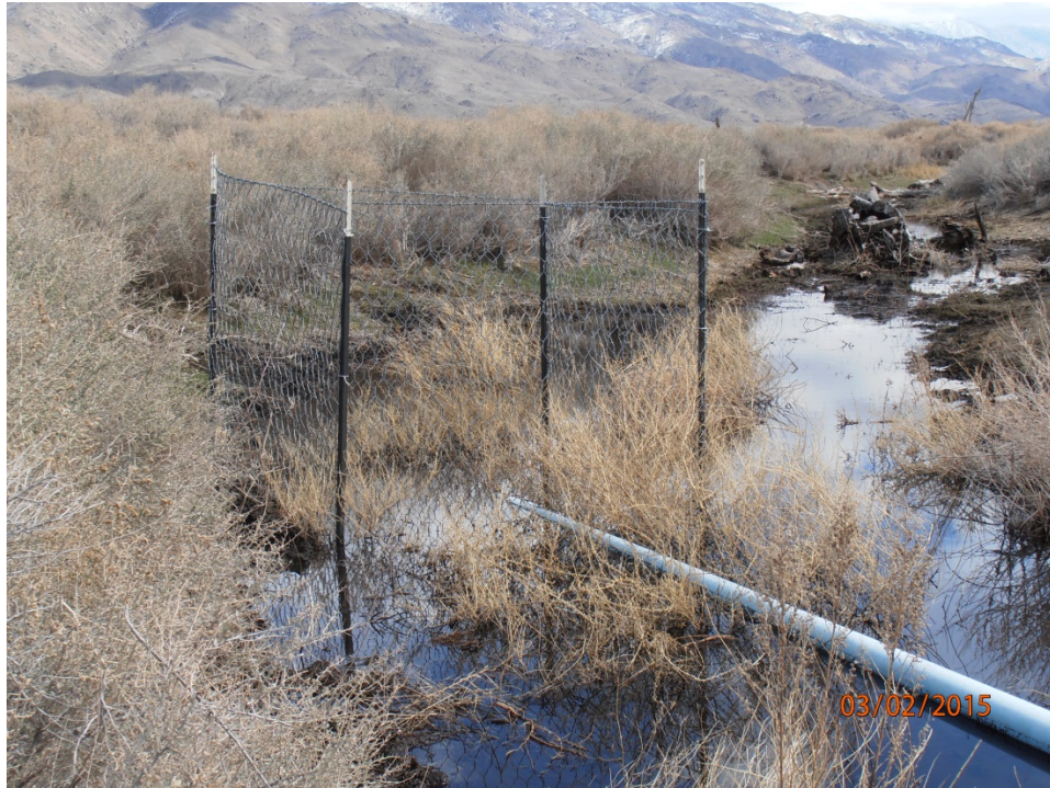
Aberdeen Channel extended outfall, March 2015.
