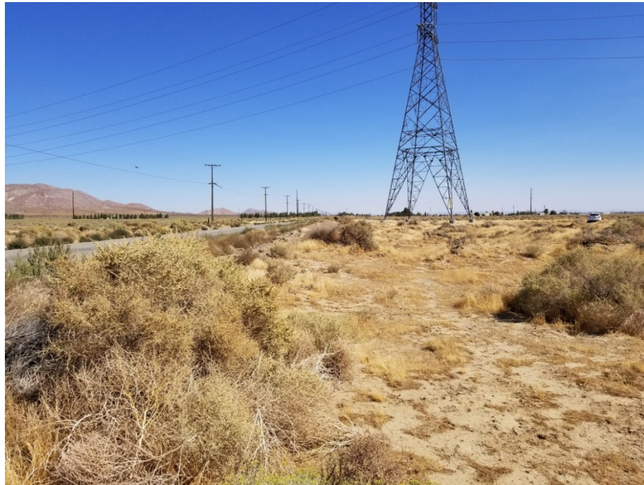
Overview of the Project site from the LADWP patrol road to the new BRRTP tower. October 6, 2017.
