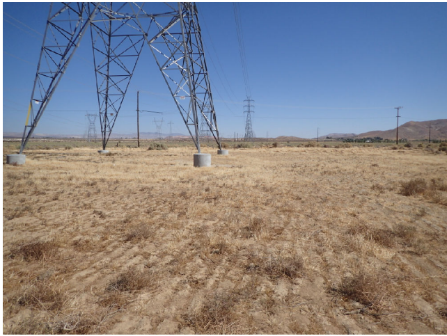
View of the transmission line towers directly west of the Project site.
