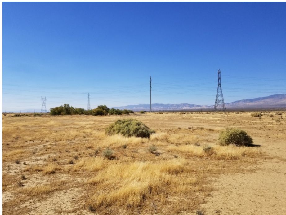
Overview of the Project site from the southeast corner of the Project site to the west. October 6, 2017.
