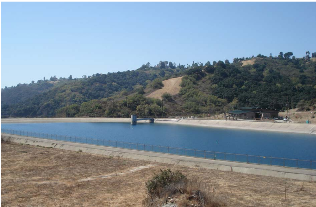
Figure 3.1-7 Upper Stone Reservoir outlet tower and chlorination station
