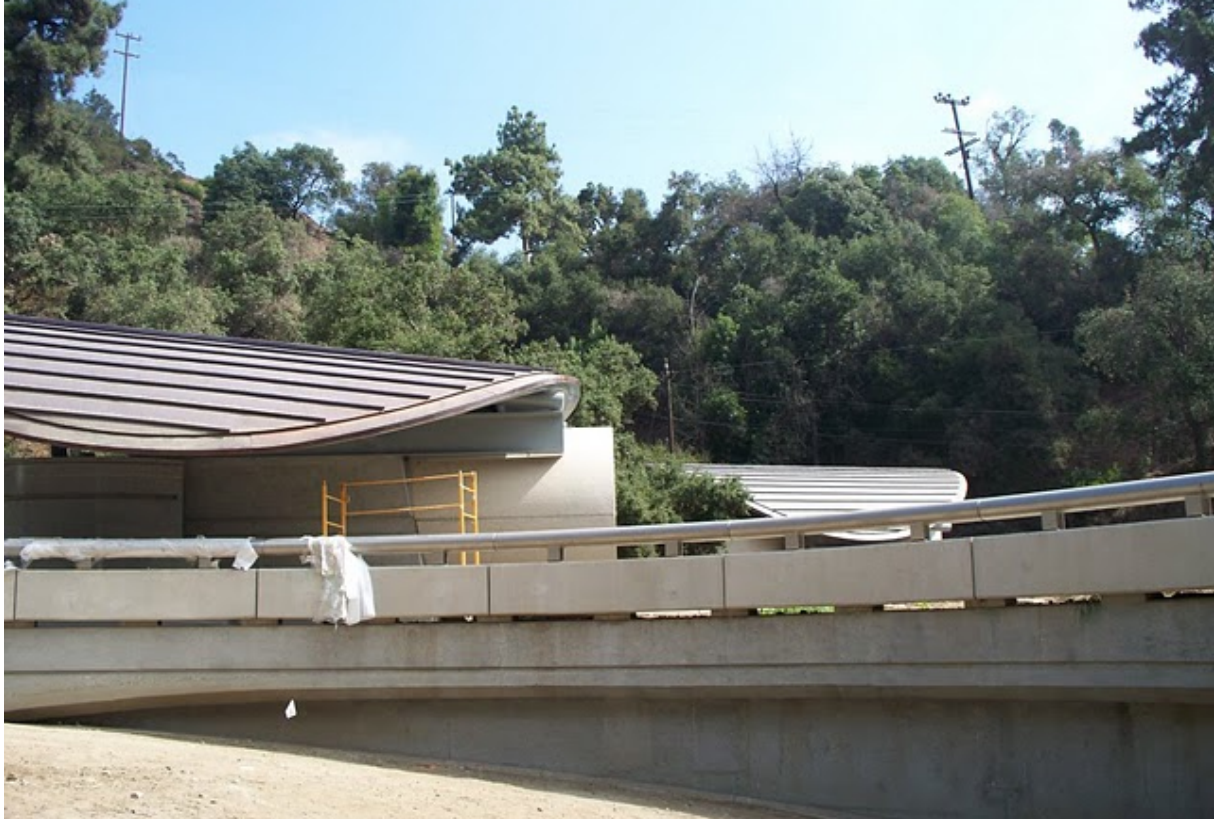
Figure 3.1-6 Lower Stone Reservoir water filtration plant
