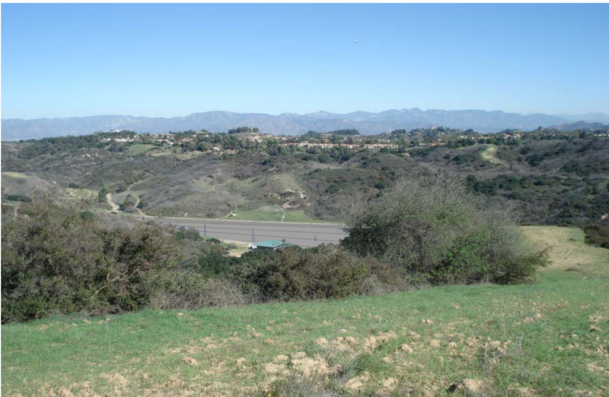
Figure 5-5 Proposed private view with floating cover from south-southwest of Upper Stone Reservoir
