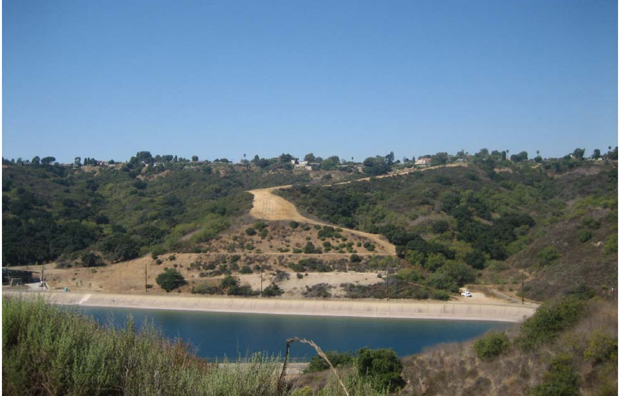
Figure 3.1-2 Upper Stone Reservoir and residential uses located on west property boundary
