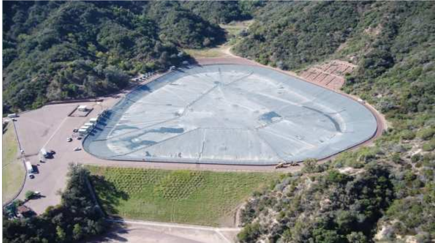
Figure 1: Santa Ynez After Installation of Floating Cover as Required by Regulation
