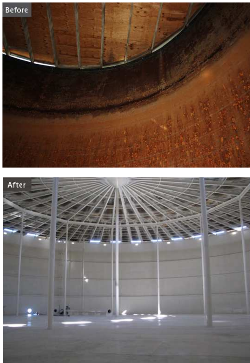
Figure 25: Water Tank Before and After Cleaning
