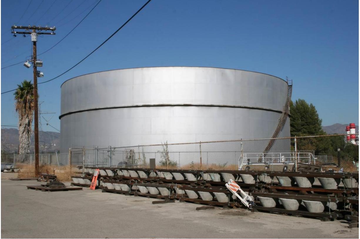
Plate 12. Water Tower, View Northwest.
