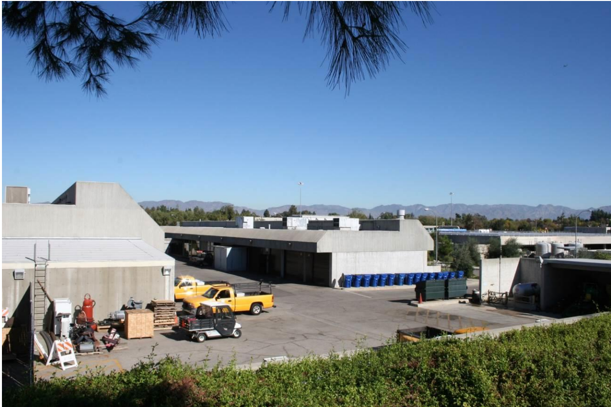
Plate 6. Donald Tillman Plant, Buildings 13 Complex in Foreground, View Northeast.
