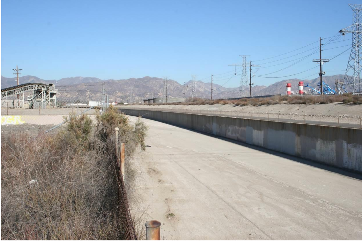
Plate 17. Tujunga Wash Southwest of San Fernando Road, View Northeast.
