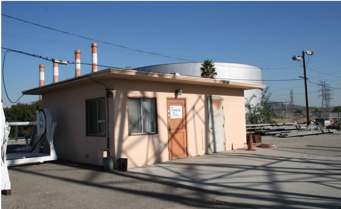
Plate 7. Building 1, Transmission School, View Southeast.
