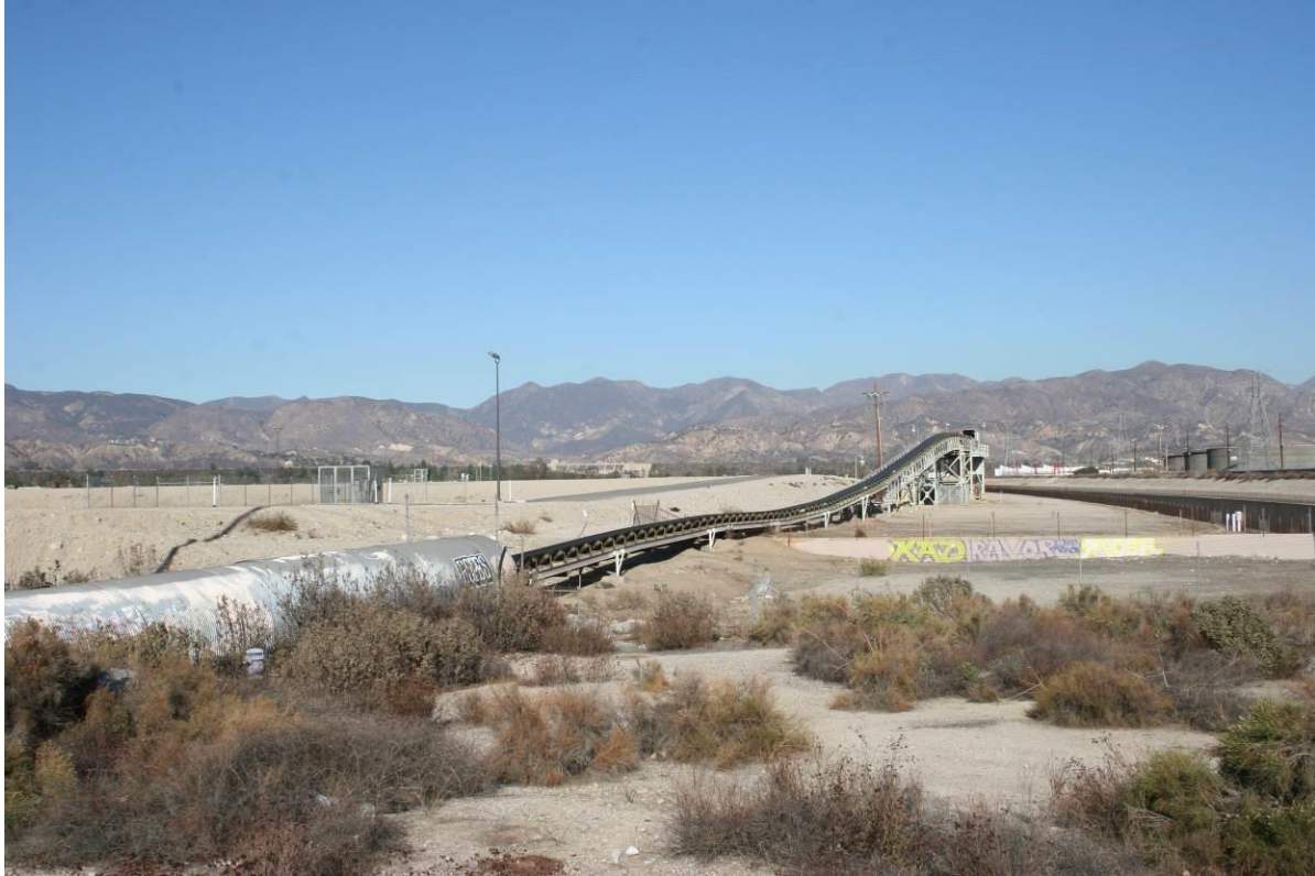
Plate 16. Conrock Co. Conveyor Tunnel Entering Hansen Spreading Grounds, View North.
