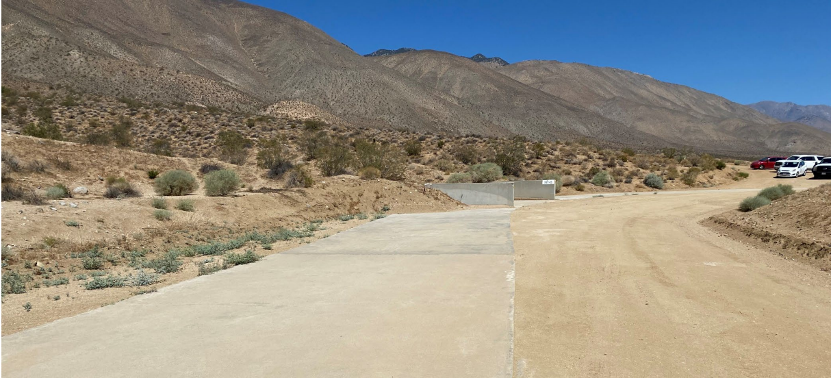
Photograph 2. First Los Angeles Aqueduct, looking north (Emily Rinaldi-Williams, Stantec June 2022).
