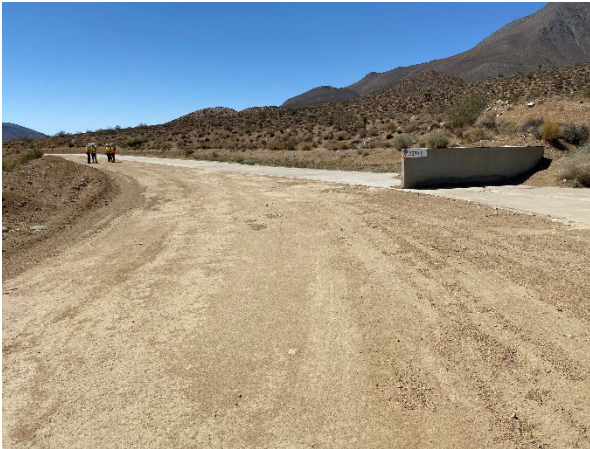
Photograph 3: Concrete wall along aqueduct, looking south (Emily Rinaldi-Williams, Stantec June 2022).
