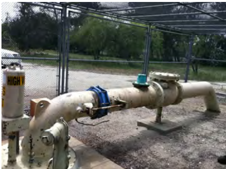
Figure 64: North Hollywood Well Site Visit
