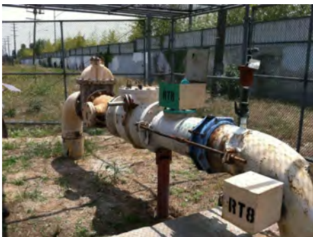
Figure 66: Rinaldi-Toluca Well Site Visit
