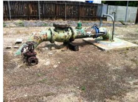
Figure 63: Erwin Well Site Visit
