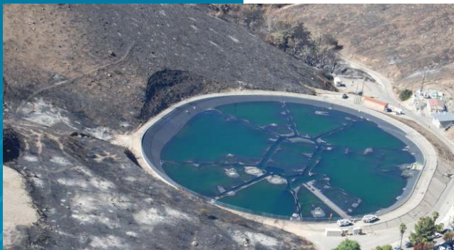
After La Tuna Canyon Fire
