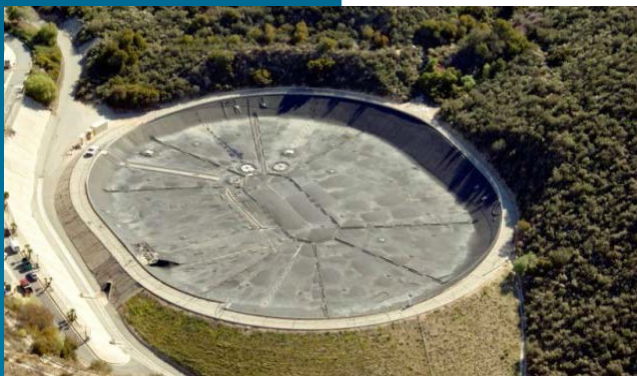
Before La Tuna Canyon Fire
